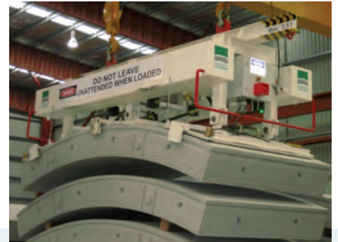
Figure 24: Safe demoulding and stacking with a vacuum lifter
