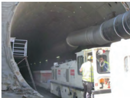
Figure 35: Portal of the TBM tunnel
