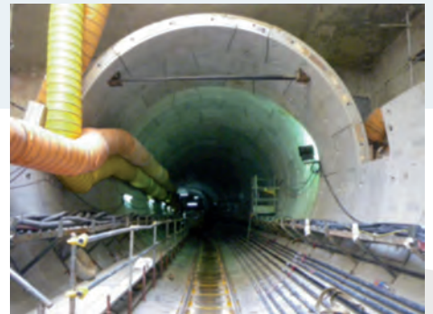
Figure 28: DTL3 C933 – View into tunnel (TBM #3)
