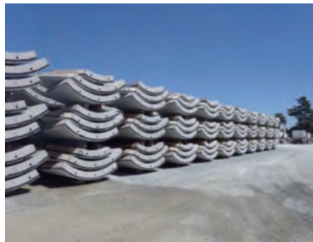
Figure 29: Project San Francisco Bay Segment production
