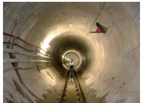
Figure 26: Project Hobson – Nearing completion
