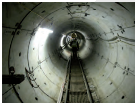
Figure 31: Segmental lining of macrosynthetic fibre reinforced TBM tunnel
