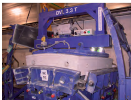
Figure 33: Demoulding of key segment
