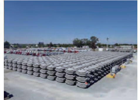
Figure 30: Segments at the production yard
