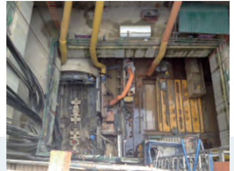
Figure 27: DTL3 C933 – East TBM launch shaft at Bendemeer station
